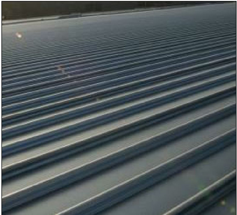
RFS-101 STANDING SEEM ROOFING SYSTEM - ROOF BLUESCOPE COLOURBOND KLIP-LOC 700 / SHALE GREY
